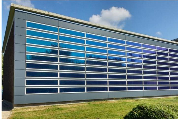
Heliatek developed the façade elements with its partners AGC and SVK. The aim of this project is to investigate the ways in which solar energy can be generated from a building facade. The installation will also allow the building integration of this technology to be tested in real operational conditions.
