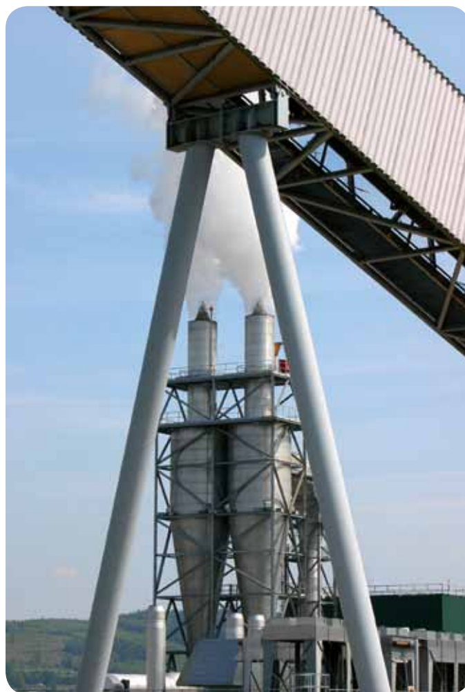
The insufficient flow generated by the fans limits the heat input and, hence, the maximum production of the dryer in the summer.
