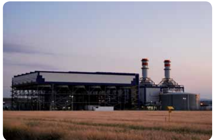
The Castelnou Power Plant relies on Laborelec's remote monitoring to identify opportunities for further improving performance.
