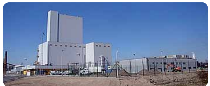
Laborelec's knowledge of European legislation was a crucial factor during the final acceptance tests of the new furnace gas power plant in Ghent, Belgium.
