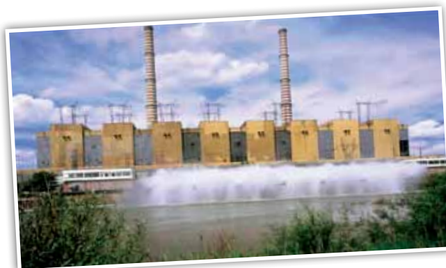
Laborelec provides extensive advice to new and existing co-firing units.
