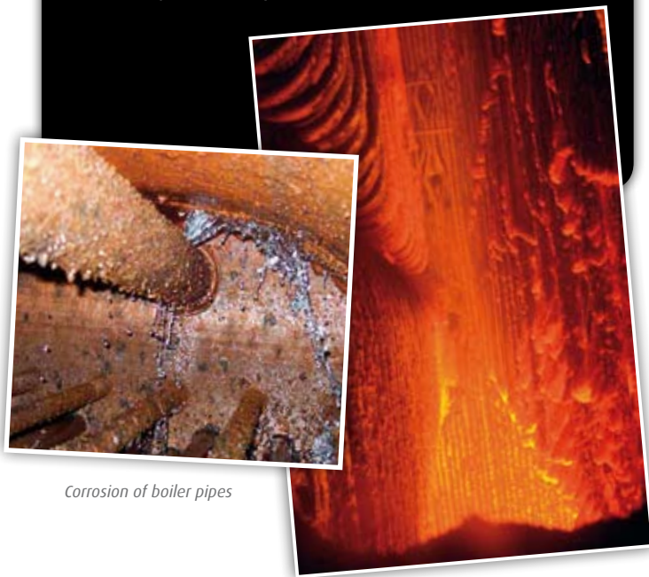
Severe slagging inside a boiler
