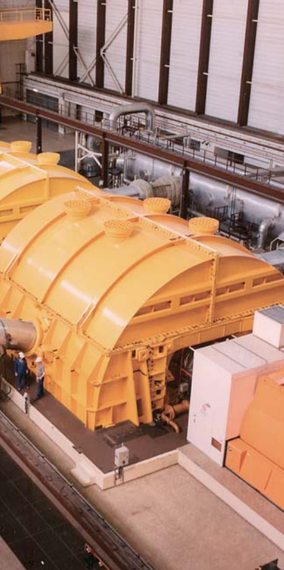
The steam turbine of the 1100 MW capacity nuclear production unit of Doel 4 (Electrabel, Belgium)
