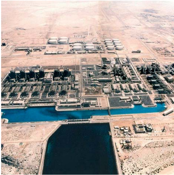
Laborelec installed a temporary LVMS system at the Al Taweelah (United Arab Emirates) facility to monitor and then analyse the data to advise them on the best solution for vibration problems at their steam turbine.
