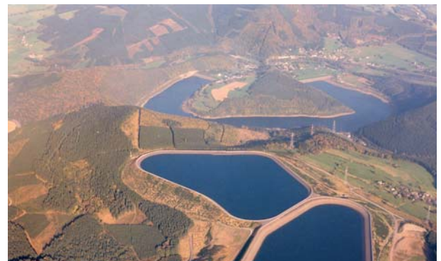
Storage reservoirs of a hydraulic power plant
