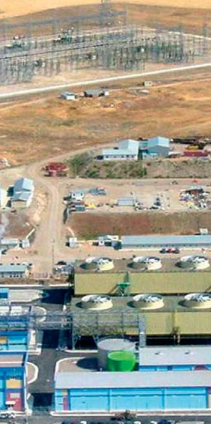
The Baymina power station is equipped with two gas turbines and one steam turbine. Total power output is 770 MW. (Tractebel (Groupe SUEZ), Turkey)
