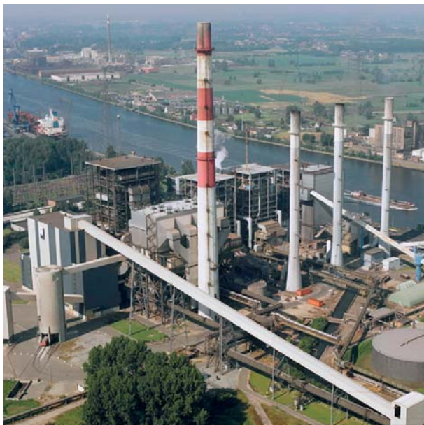
The Rodenhuize power plant has had a very cost effective LVMS assistance contract with Laborelec since 1985.
