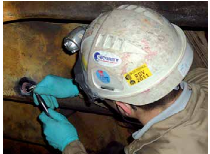
On-site replica inspection
